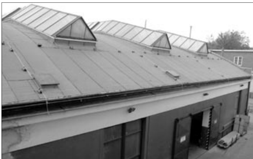
Reconstructed WEMA buildings still exist in Prague. The rooflights and supporting roof construction have not changed even after three quarters of a century
